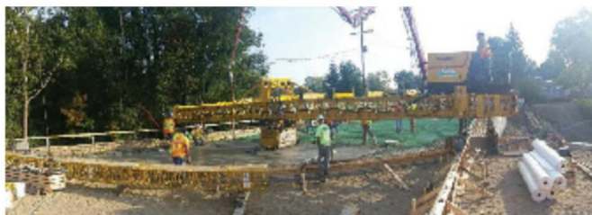
Plasterers and Cement Masons pour a bridge near Frankfort, IN.
