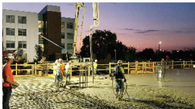
Plasterers and Cement Masons pour a floor at the Flex Lab Facility at Purdue University.
