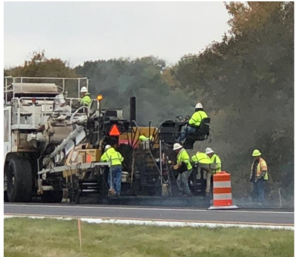
Paving crew road resurfacing
